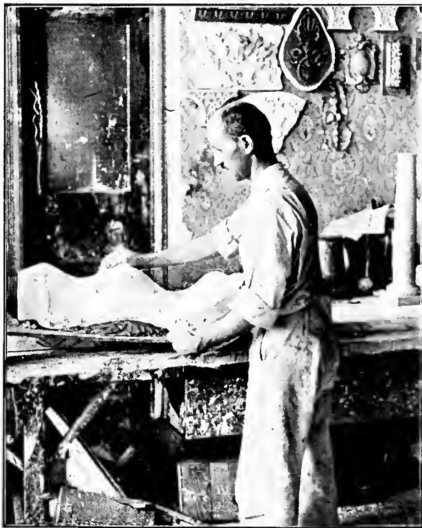
Fig. 64—Plaster Case being Cast on Model over Clay
